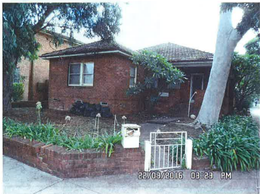
View of 13 Hornsey Road (the Rectory site)
